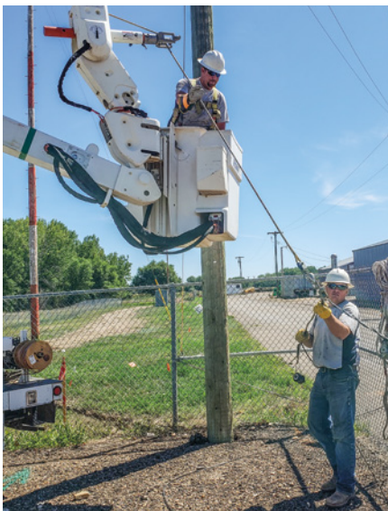
Lower Yellowstone Rural Electric Cooperative lineworkers Tanner Roth (in bucket) and Lee Alvstad upgrade the electric service at the Sidney-Richland Airport. The two-way feed will assist in minimizing outage times at the airport and surrounding areas.
