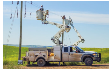
The LYREC crew replaces a pole and cross arms during the July 8 planned power outage.
