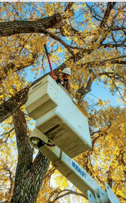
Journeyman lineworker Tanner Roth saves a kitten that had been stuck in a tree for three days.
