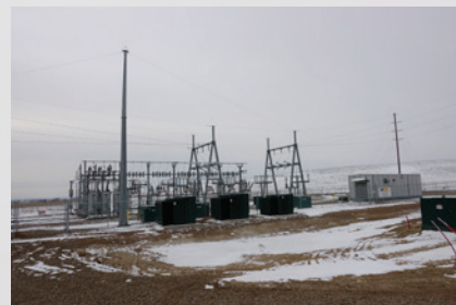
Completed construction of two substations. The Iversen Substation was energized in August and the Helmut Substation was energized in October.
