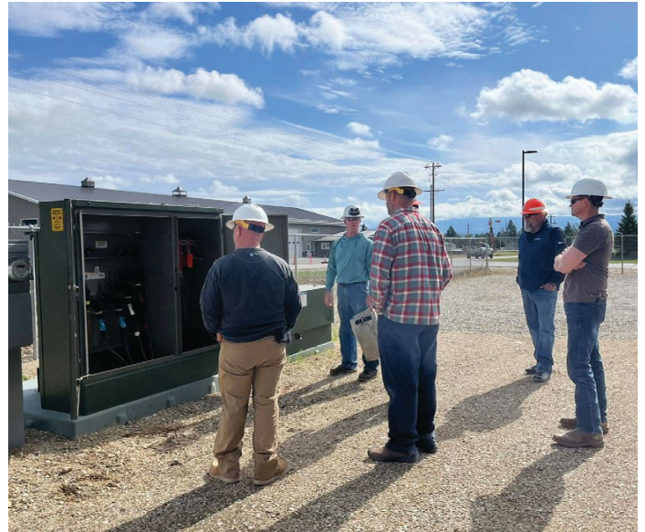
Montana electric cooperative staff complete safety evaluations at Ravalli Electric during a recent RESAP inspection. | REC PHOTO
